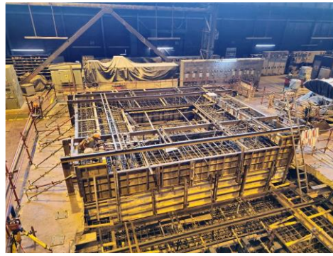
Plate Mill Main Drive base demolition and reconstruction
